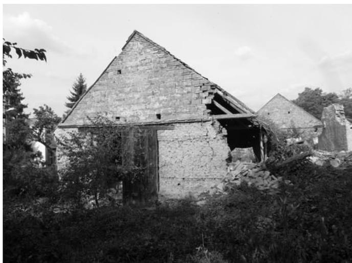
Figure 7. Remains of barn built with coffered *války* in Míšovice (distr. Znojmo) (Credits Zuzana Syrová 2016).
