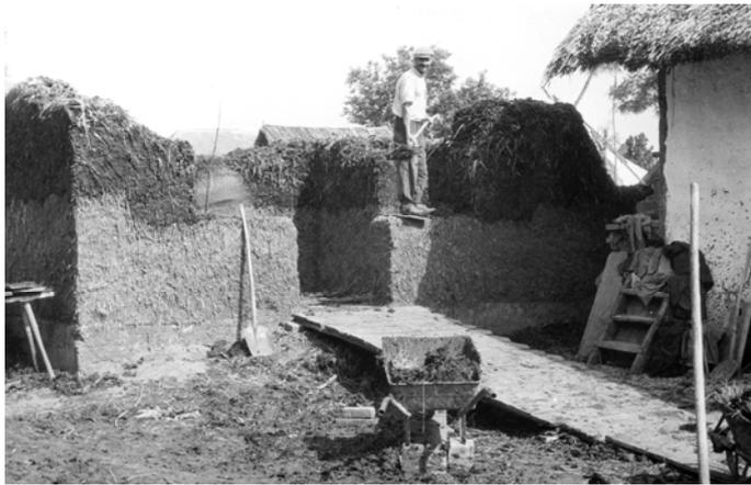
Figure 1. 3.1 Pitched-forked cob construction in Žitný Ostrov (Rye island) in 1950s (Credits Václav Mencl)
