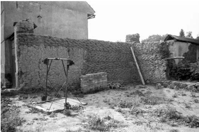
Figure 4. *Války* structure of the remains of cottage with partially conserved plastering of interior surface of the walls and visible piece of wood that served as reinforcement of its corner; Hruška (distr. Prostějov) (Credits Zuzana Syrová 2000).
