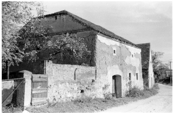
Figure 2. Wine cellar built with pitched-forked (?) cob in Šatov (dist. Znojmo) (Credits Zuzana Syrová 1995).
