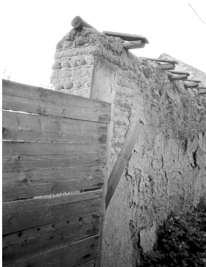
Figure 6. Remains of the barn built with cylindrical války in Hruška (distr. Prostějov) (Credits Zuzana Syrová 1995).
