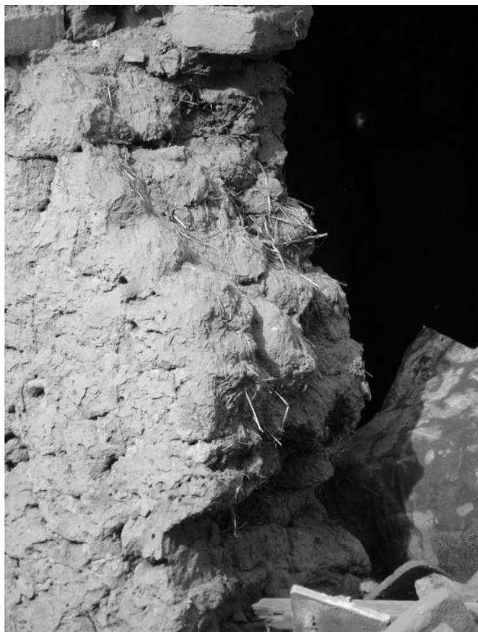
Figure 8. Detail of the cob structure of the Míšovice barn. (Credits Zuzana Syrová 2016).
