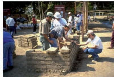
PAT 96 course participants construct an adobe wall near the archaeological site of Huaca del Sol in the Moche Valley, La Libertad, Peru. Photo: Leslie Rainer, GCI
